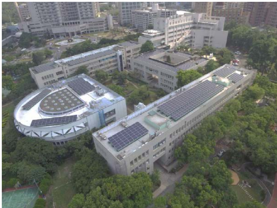
Figure 2 The first phase of installation of the solar photovoltaic power generation equipment
